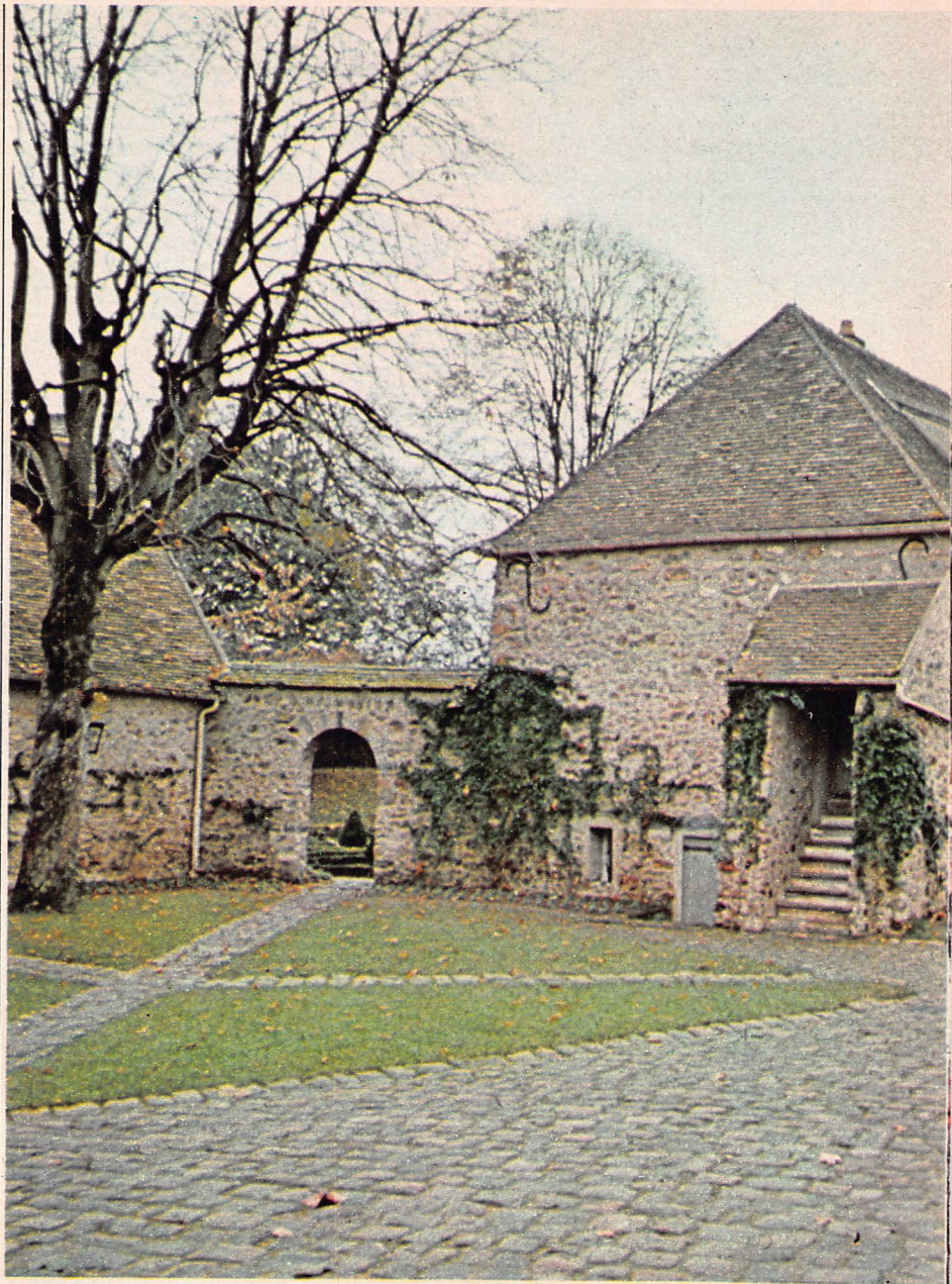
Part of the main house.
